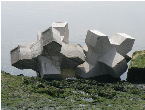
Figure 17: X-blocks used in Ijmuiden for placement of eco-slabs (Ecoshape, sd).
