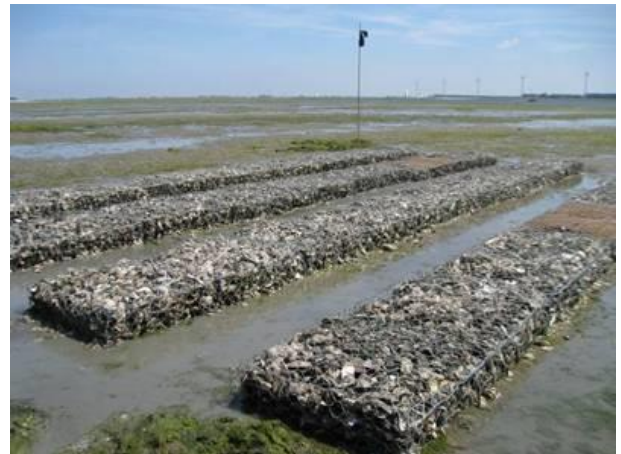
Figure 13 Gabions filled with oyster shells provide a substrate for new reef formation.
